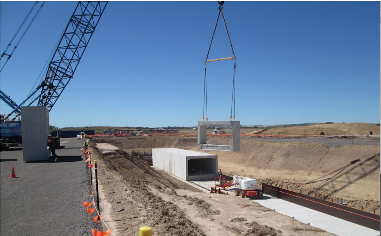
Figure 1 – Train Load Out Development In Progress
