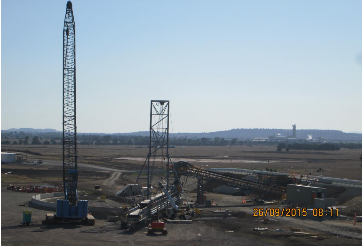
Figure 2 Train Load out Development in Progress
